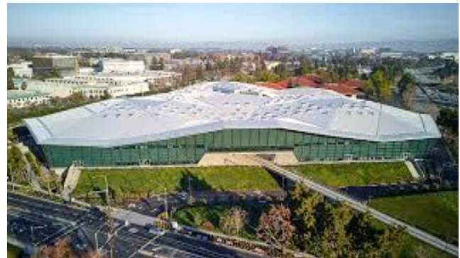
NVIDIA Headquarters, Santa Clara, CA
